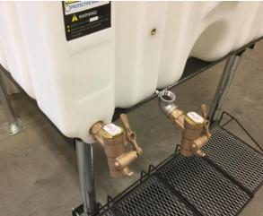
8. Install Poly Elbow(s) 90 Deg PP 1" MNPT X Hose Barb (P/N: RTT-4003) into stacked tank drain port(s). Angle poly elbows at a 5 o'clock position, aiming to its corresponding stand elbow kit. Repeat as necessary NOTE: All threaded fittings must be coated with sufficient pipe thread sealant to prevent leakage. RTT recommends Gasoila Thread Sealant (P/N: RTT-4031).
