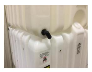
**9.** Install Poly Union(s) Adapter PP 1" MNPT X Hose Barb (P/N: RTT-4004) into Stand Elbow Kit(s). *Repeat as necessary*NOTE: All threaded fittings must be coated with sufficient pipe thread sealant to prevent leakage. RTT recommends Gasoila Thread Sealant (P/N: RTT-4031).
