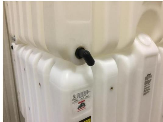
9. Install Poly Union(s) Adapter PP 1" MNPT X Hose Barb (P/N: RTT-4004) into Stand Elbow Kit(s). *Repeat as necessary*
