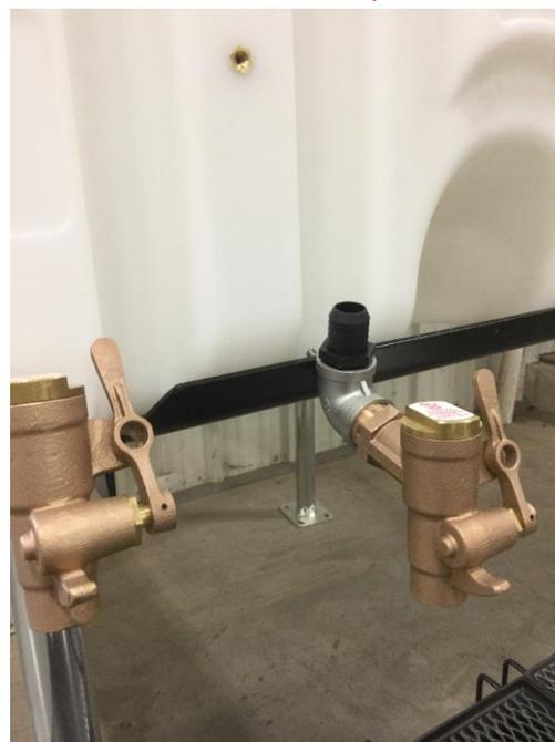
10. Cut to length and attach Braided Poly Tubing (P/N: RTT-4009) to barbed ends of the Poly Elbow(s) and Poly Union(s)
