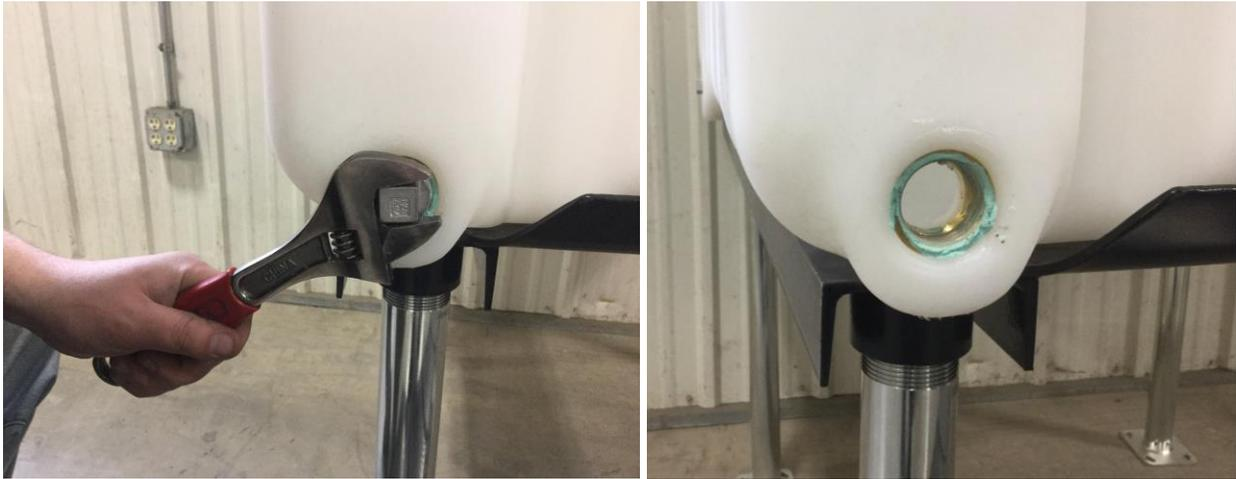
7. Install 1" Brass Spring Release Valve (P/N: RTT-4001) directly into bottom tank drain port. Install additional Valves into Elbow Kits on Stand. Be sure to support the Elbow Kit so as not to put unnecessary pressure on the Elbow Kit Bolt.
